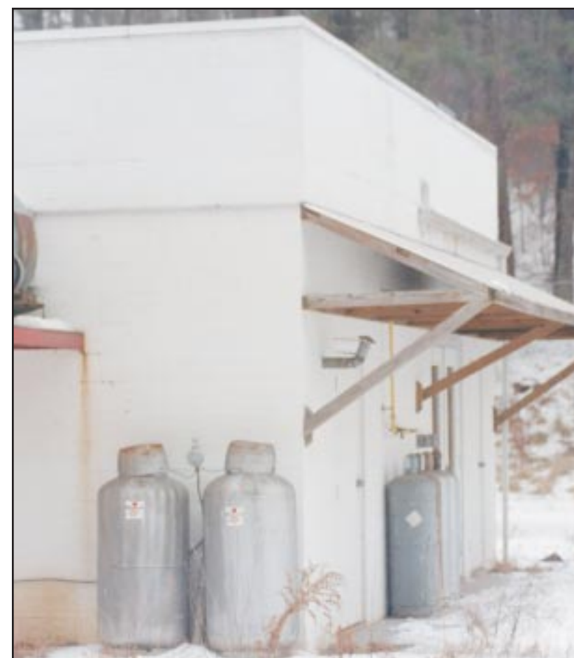
Tanks are stored outside of the structure used to practice firefighting skills. This building is located on Penn State property, relatively near drinking water wells.
